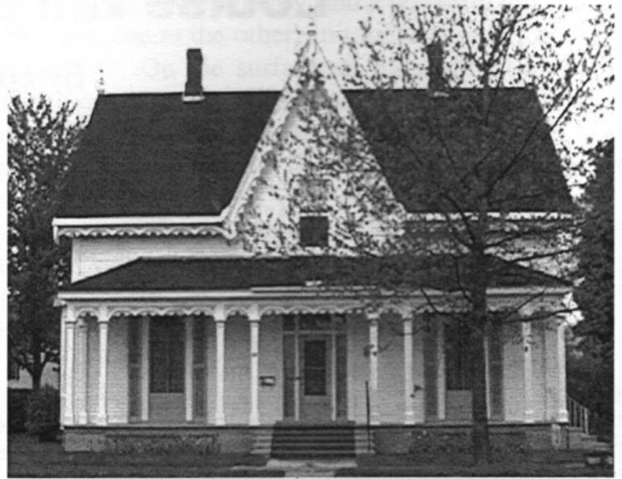
92 Waterloo Row Front View
