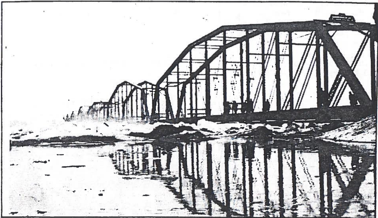
DOOMED BRIDGE - Frank Pridham of Harvey Studios got this last photo of the doomed railway bridge in the early afternoon of March 19, 1936.
