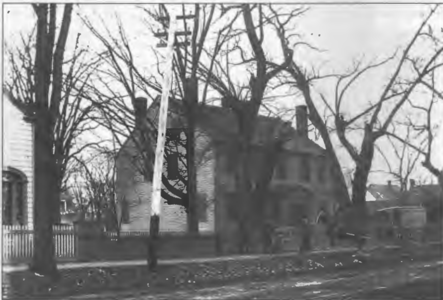
Edgcombe House. A photo from the George T. Taylor Collection, showing the original structure. (Photo courtesy of the Provincial Archives of New Brunswick.)
