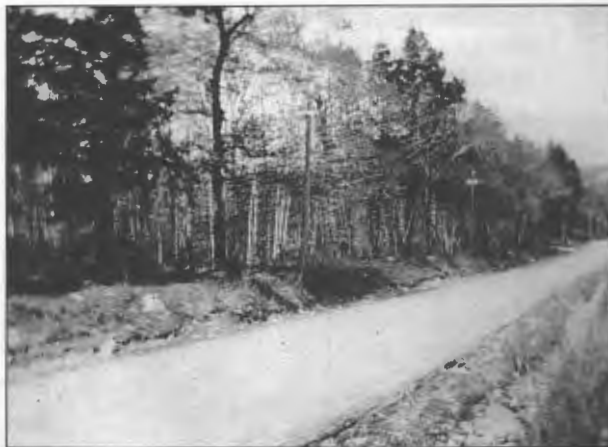
New Maryland Highway Road, c. 1930. (Photo Courtesy of Margery Squires Acheson.)
