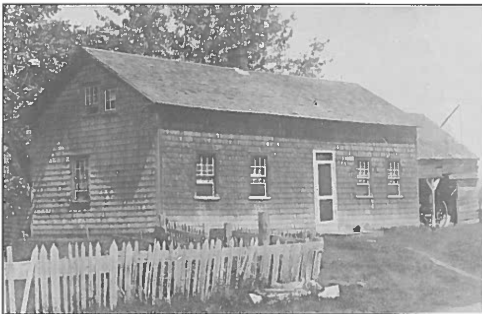
This 1810 house in Zealand, where Oscar Morehouse was born, was demolished in 1960.
